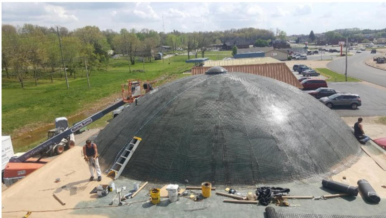
(above, a “dome” covered with basalt fabric: This dome is a product of basalt fibers: **great for shielded structures** housing many otherwise unshielded habitats, but also for factories and sports arenas)
